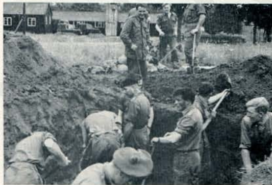
Devizes, July 1965— Digging the Battalion Command Post
