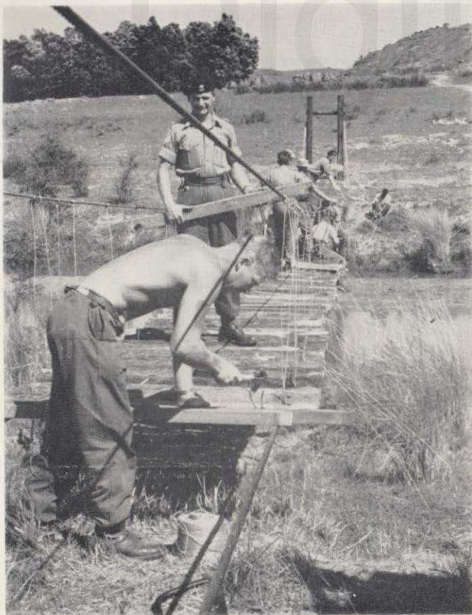
A 75 yard span suspension bridge being built by the Assault Pioneers over the Umbulzi River in Swaziland
